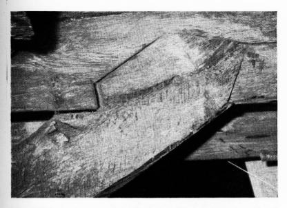
FIG. 8. The lower of the two notched-laps in the belfry, here designed to withstand mainly compression, but also notched to resist any tendency to withdrawal.
