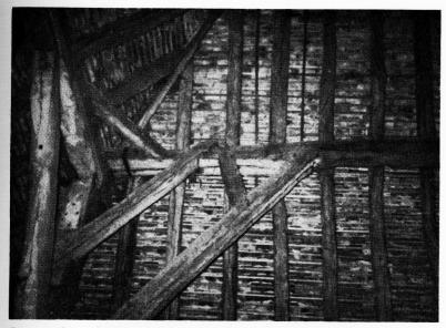
FIG. 10. The south-eastern end-frame post, showing that all transverse braces are either notched or lapped, whilst longitudinal braces appear to be tenoned.
